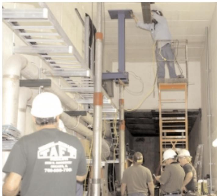
Contractors supervised by lab personnel are installing the first 29 magnets of the new NuMI beam line.
