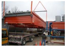
A 30-ton cooling tower for CHL is unloaded from a tractor trailer prior to installation.
