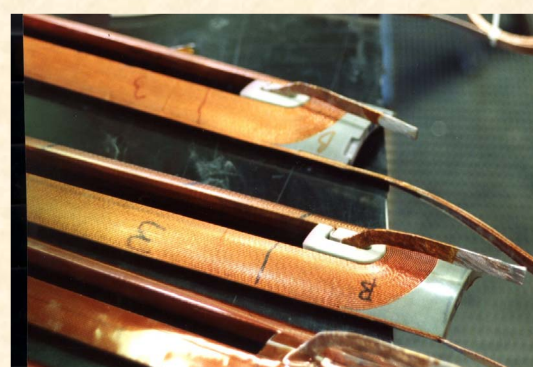
LBQ coils during construction.
