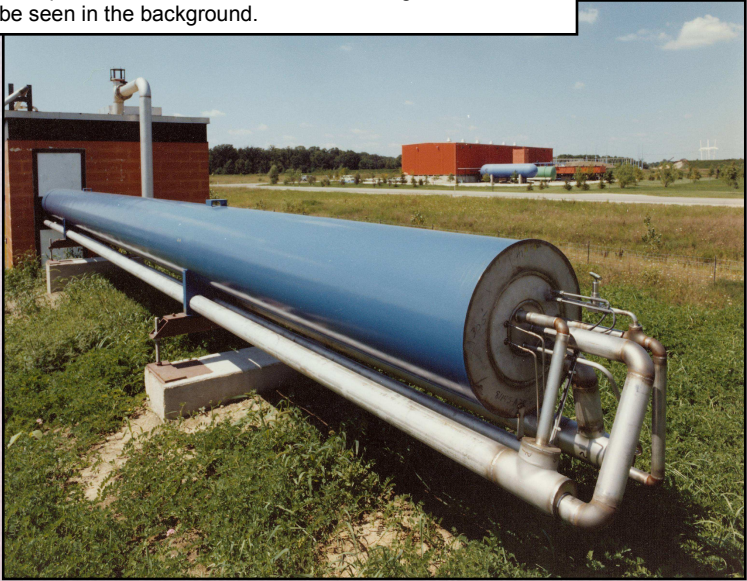
Tevatron Satellite Refrigerator Heat Exchanger: Each satellite refrigerator incorporates a horizontal spiral wound, finned tube heat exchanger. The Central Helium Liquefier can be seen in the background.
