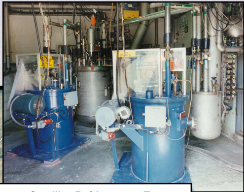
Tevatron Satellite Refrigerator: Twenty-four satellite refrigerators, each with a capacity of 1kW at 4.5K, are spaced around the four mile accelerator. Two reciprocating expanders are shown.
