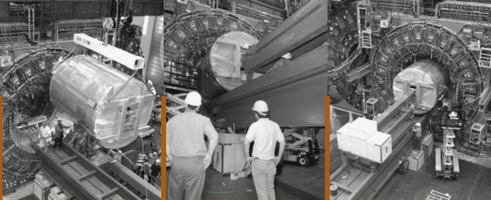
The COT is lowered into position on the siege cart (left). Mukherjee likens the siege cart (center) to a “battering ram,” but its job is to coax the COT into the center of the big CDF detector (right). Technicians stationed inside the big detector (below) guided the COT into position with only two millimeters of radial clearance. They were able to make adjustments in both the siege cart and the “H-frame” to avoid contact.
