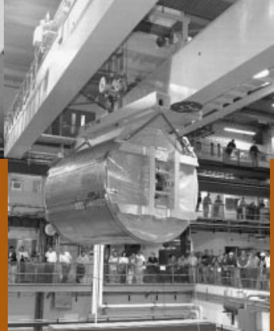
The truck trip took about half an hour (left), with the COT mounted on the same stand used for assembly in IB4. Project co-leader Aseet Mukherjee explained that the wheeled support would allow the “can” to roll in accommodating any flexing by the truck bed. The COT was then lifted by crane (right) into the CDF Assembly Hall.
