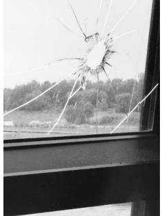
Falling concrete punctured this hole in a south-facing window.
