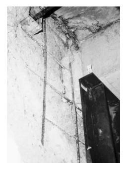
Seasonal stresses on structural beams have exposed these steel support rods in the concrete.
