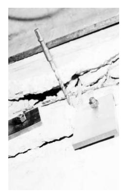
Reinforcing plates hold loose pieces of concrete in place.
